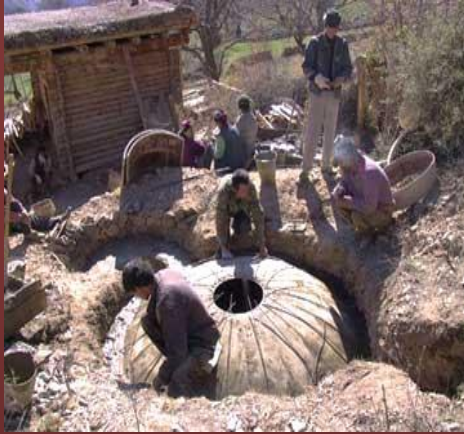
Biogas: generation of electricity from human and animal waste
