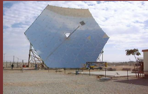
PETAL (photon energy transformation astrophysics laboratory) for the generation of solar electricity
