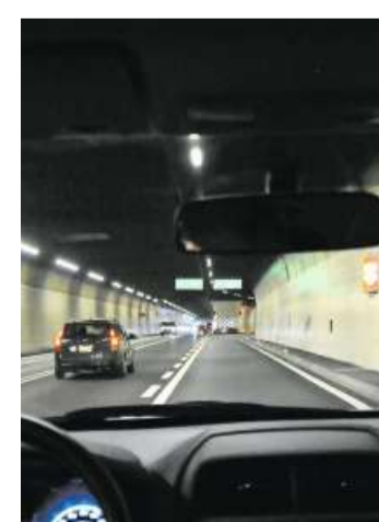
Blick in den Tunnel Lopper.
